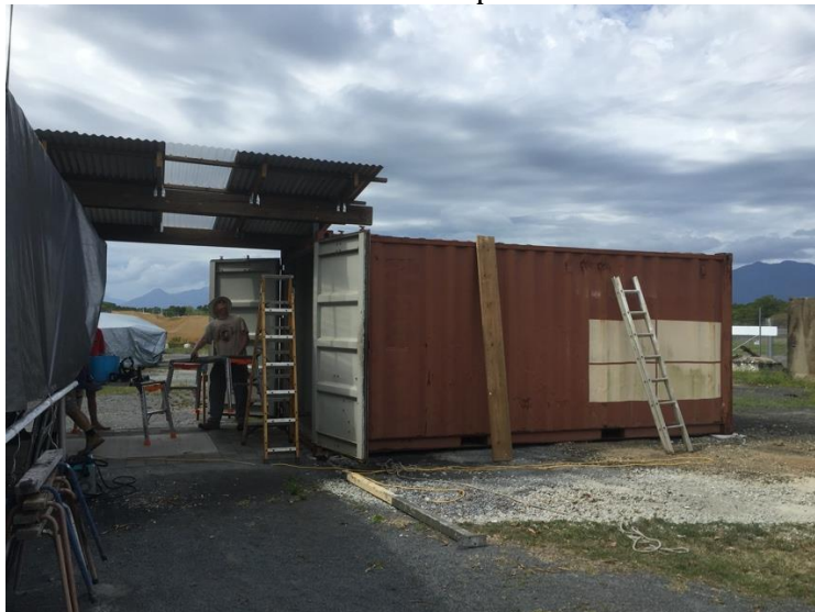
Roof attached, and complete, again.
