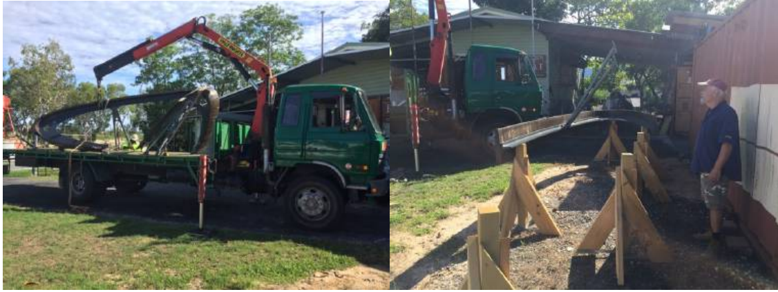
Brendon supervising the lift, first frame in position.
